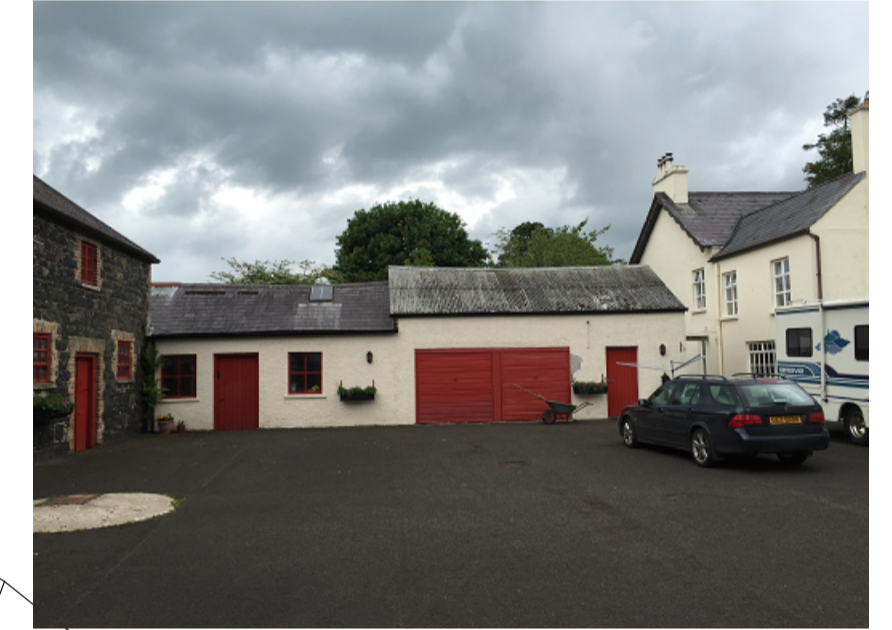
Outbuildings around the Courtyard.
