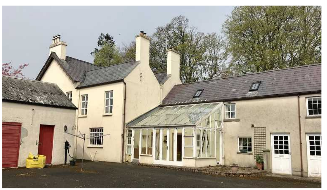
View of Currysiskan House from Courtyard.
