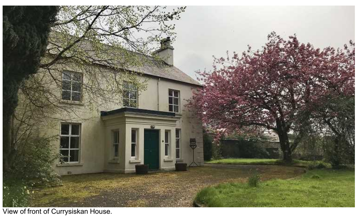
View of front of Currysiskan House.
